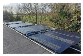
We've taken another small but important step to a <u>net zero NHS</u> at our Bainbridge and Preston ambulance stations. The old oil system has been replaced with solar photovoltaics (PV), supporting a thermodynamic heating system at both sites which will provide solar heating to the ambulance stations. Compared to oil, the thermodynamic heating system provides the same thermal output at half the running cost and with an 84% reduction in carbon emissions.
